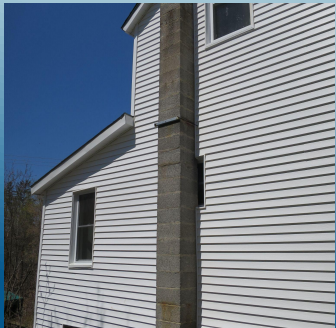
After: new siding = new house!
