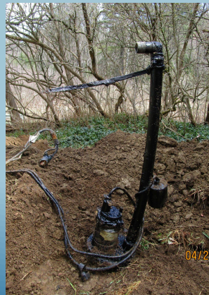
Before: Emergency replacement of septic pump
