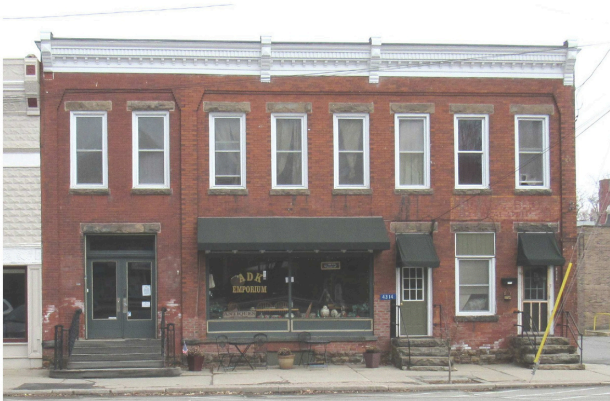
Front View, existing conditions, March 2018
