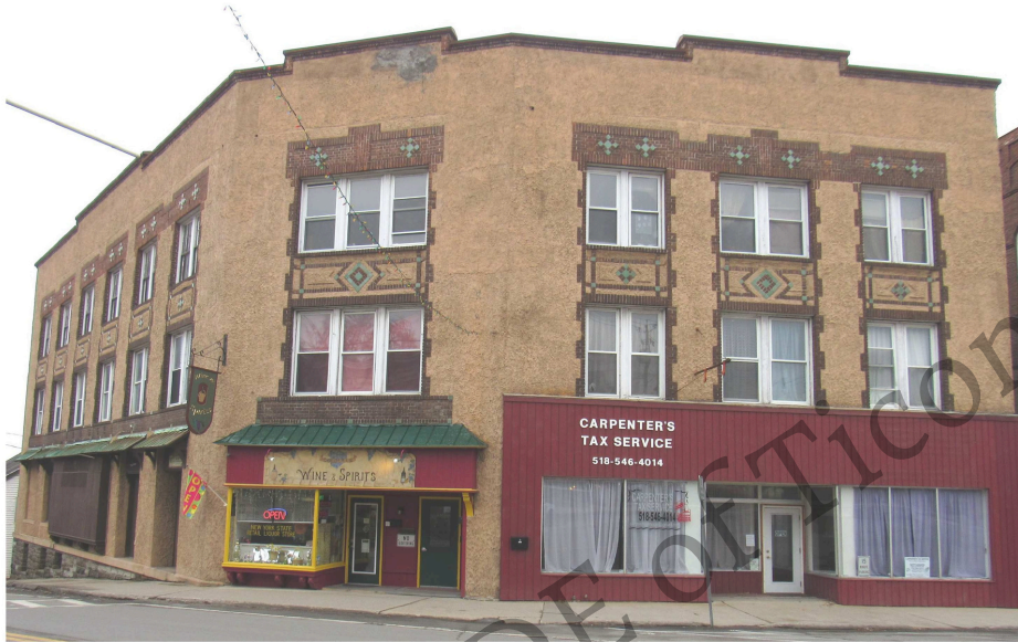
Existing Conditions – March 2018 – Foote Block, Celotti's Wine Store
