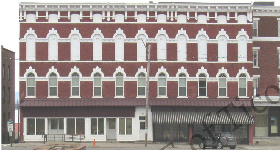
Mountain Lake Services Building, also known historically as the Van Orman Block
