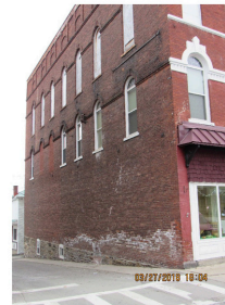
Alley elevation – masonry repairs
