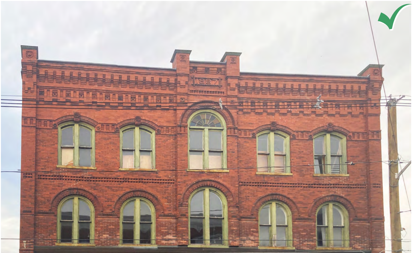
Restore and repair original wood windows whenever their condition warrants it. To provide additional thermal protection, new interior storm windows can be a cost effective alternative to replacement windows.
