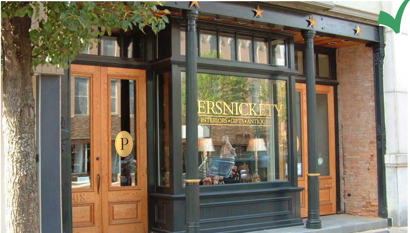
Use and maintain wood details when appropriate, such as at storefronts, windows, and doors.
