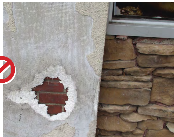
Do not use EIFS to cover original materials or in places requiring durability.
