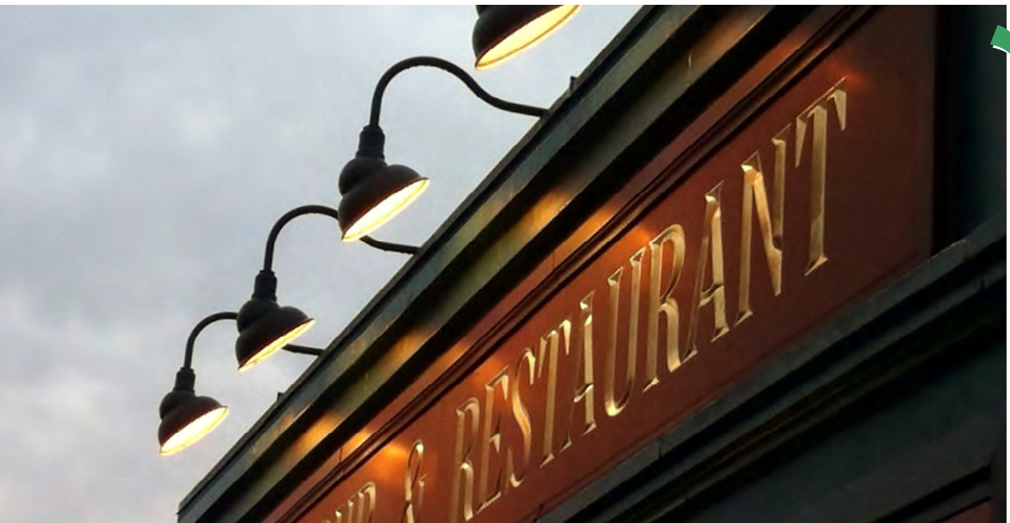
Space fixtures apart to create an even level of lighting across a signboard.
