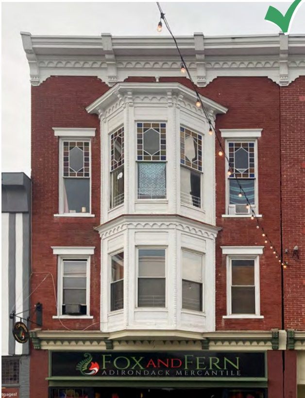
When still in tact, restore and repair existing millwork.
