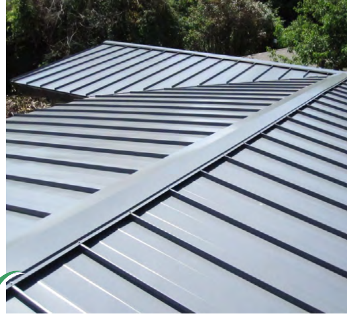
A standing seam metal roof will make a great, long lasting replacement.
