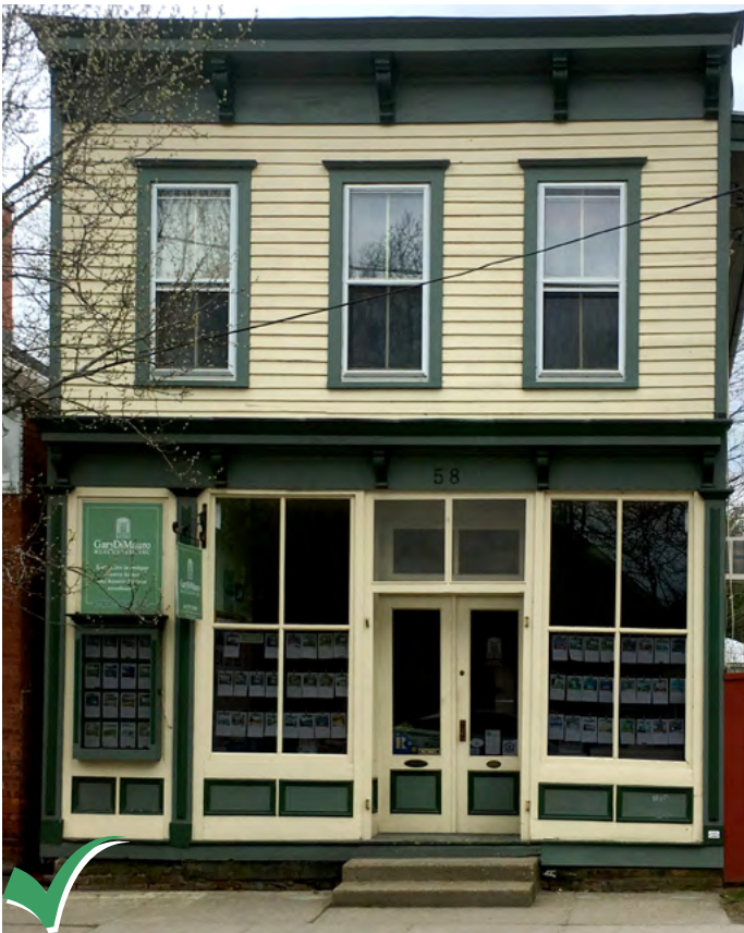
Use contrasting colors on your siding and trim to highlight details unique to wood construction.
