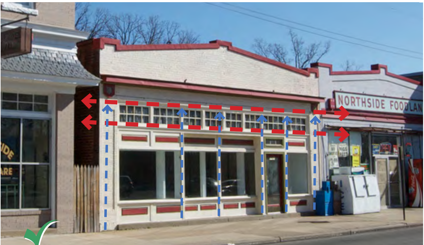
Use transom windows to add horizontal lines that break up the height of window openings.
