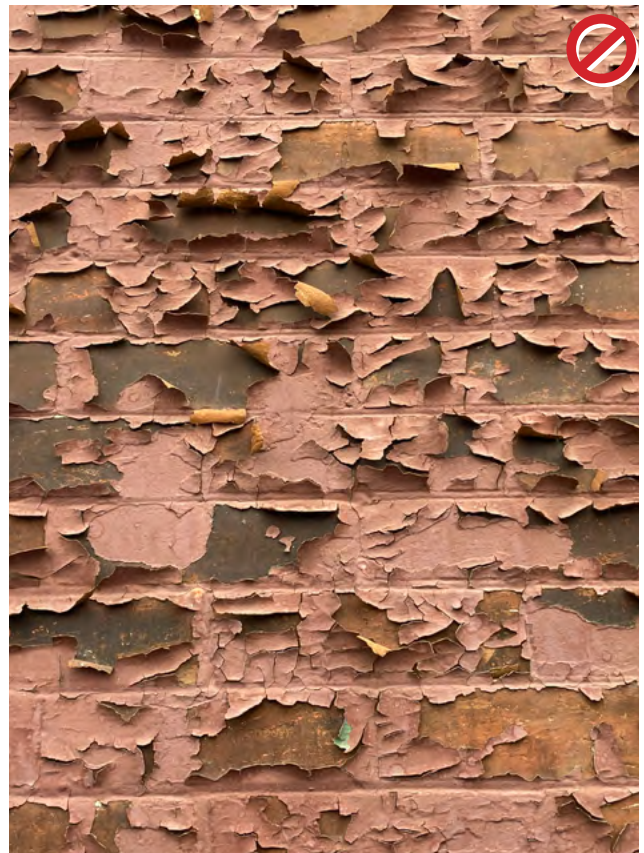
Don't paint historic masonry, it seals moisture in the material and will inevitably cause peeling.
