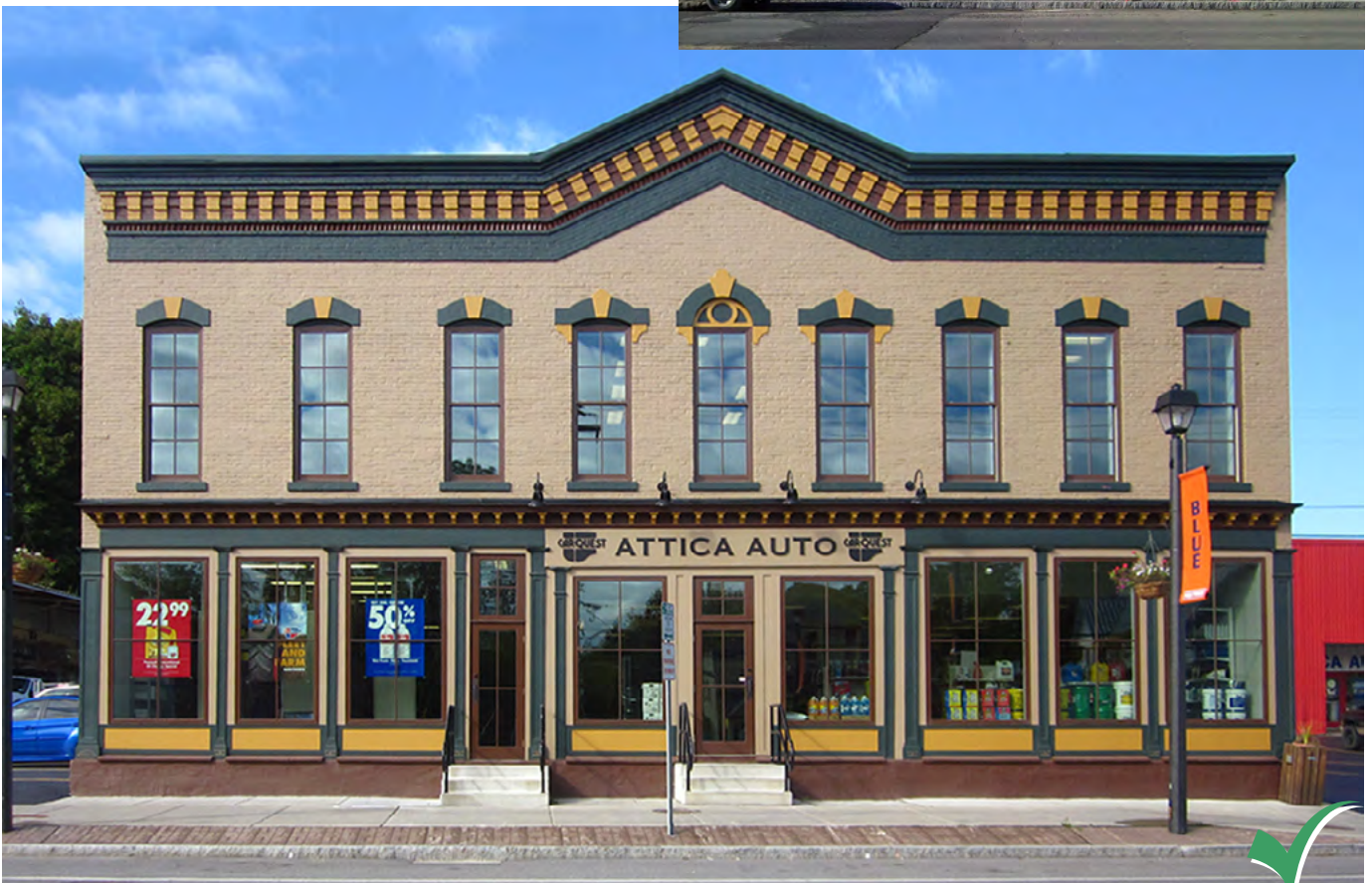
Restore original window openings that have been covered up over time. Highlight original masonry details with contrasting paint color schemes.
