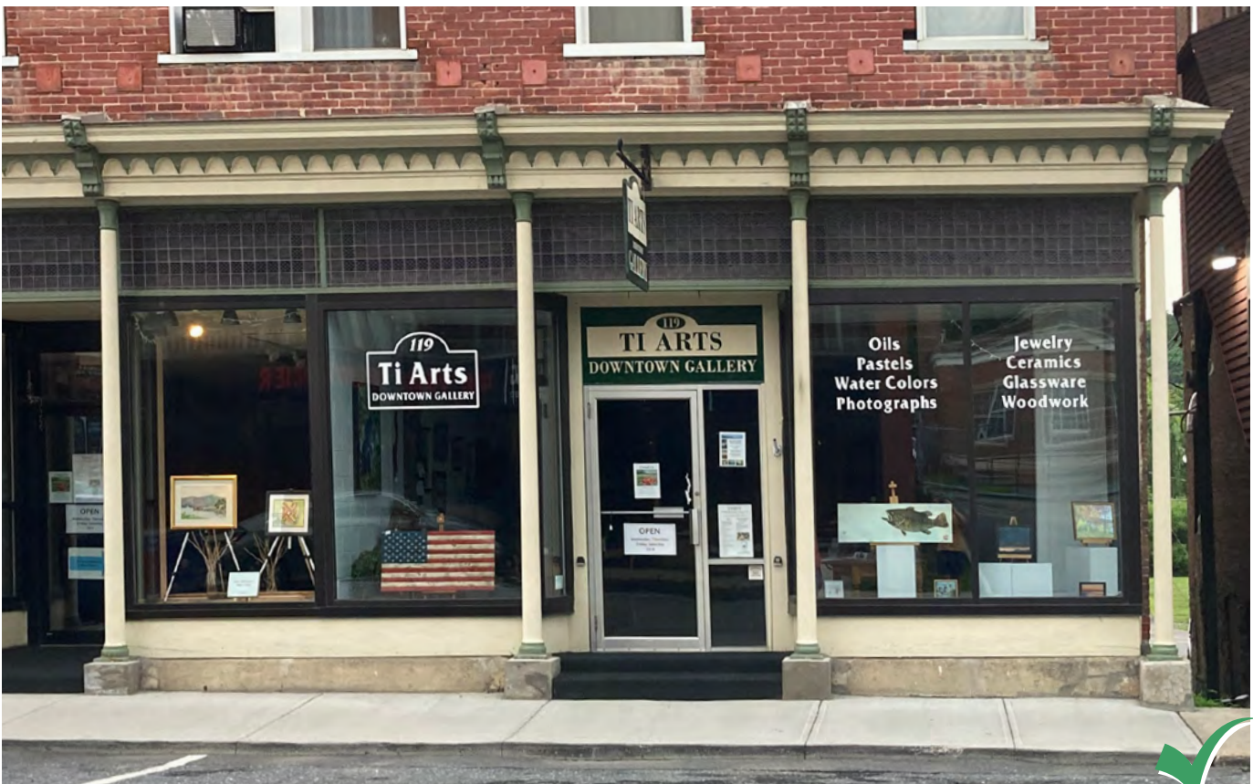
Original steel columns and cornices can be uncovered and restored to provide authentic character to a storefront.
