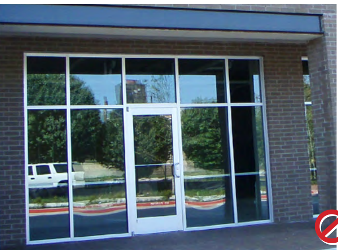
Do not use floor to ceiling tinted glass or prefabricated metal storefronts
