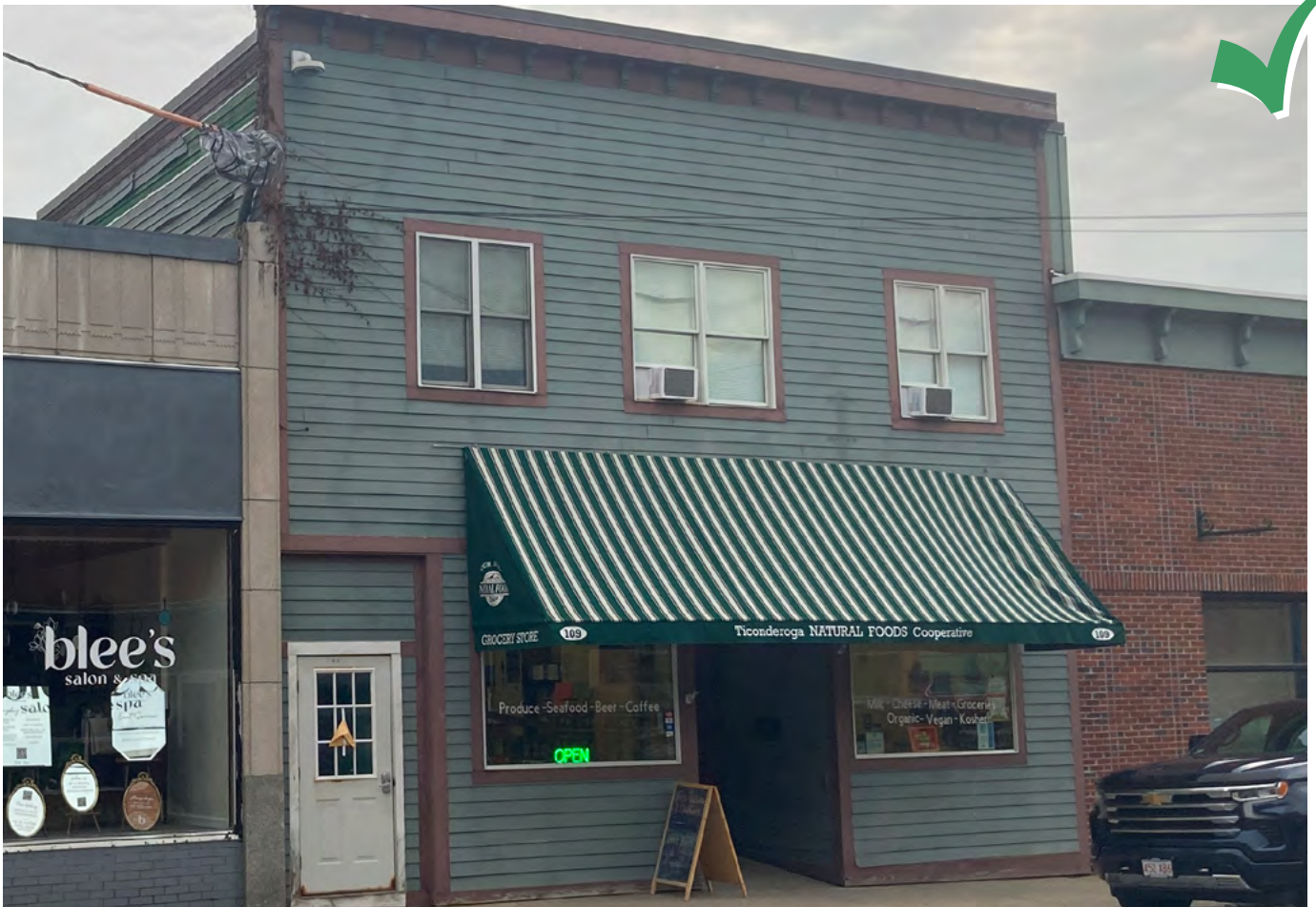
Use materials that can be repaired and maintained similarly to the original - such as fiber cement in place of wood where durability is desired.
