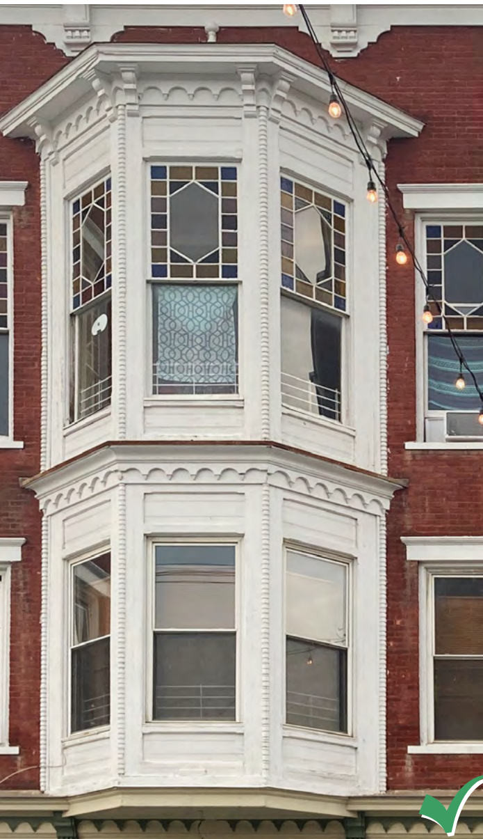
Historic oriel windows can have a long lifespan if properly maintained.
