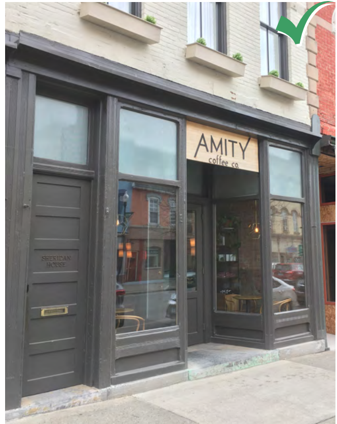
Commercial and residential entries should be different enough to distinguish their use.
