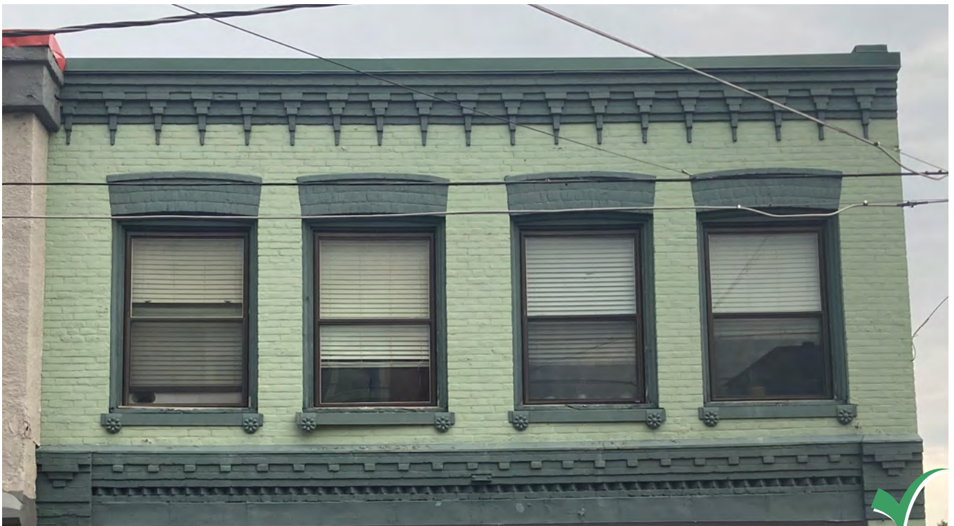
Restore and maintain historic masonry detailing, and accentuate it with color.
