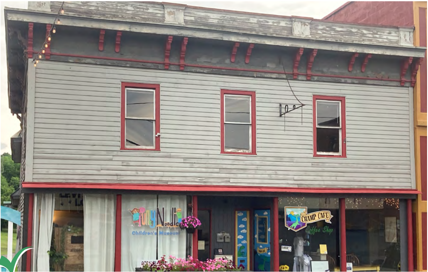
Maintain and restore original wood siding and millwork through periodic scraping and repainting, with damaged elements replaced with similar materials.
