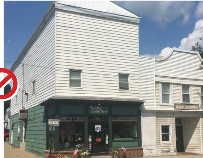
Do not use vinyl or metal siding to cover up facade detailing and depth.
